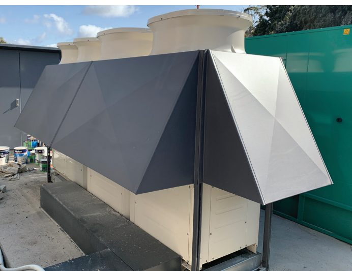
CITY MULTI outdoor units fitted with snow hoods
