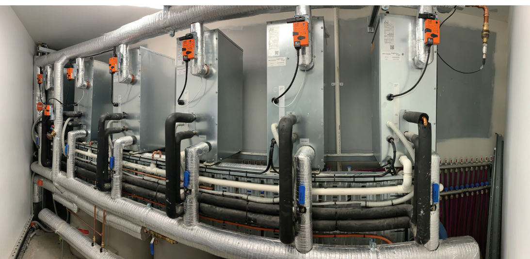
CITY MULTI PWFY HEX (Heat Exchanger) units.
